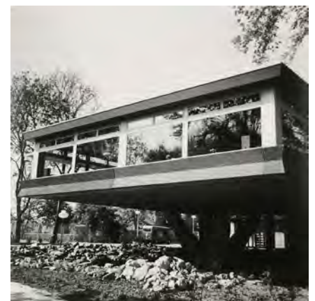
Shell canteen (1976) featuring cantilevered concrete structure and gravel concrete floor belts.
