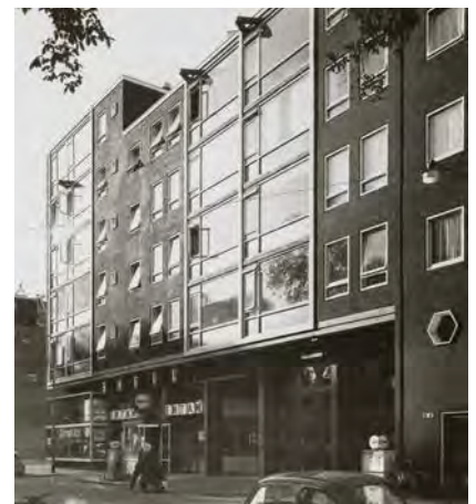
The Waterlooplein-complex (1966) showing ground level with Shell service station, garage and a Ford showroom, of which nothing can be found now.
