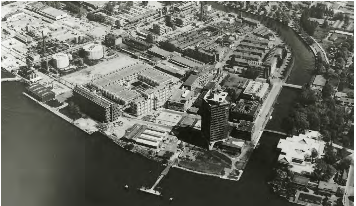
The Shell technology campus with the Shell tower in front and the Shell canteen on right the north banks of the IJ river (1976). Image: Sandra Guarda The Importance of Being Overhoeks .
