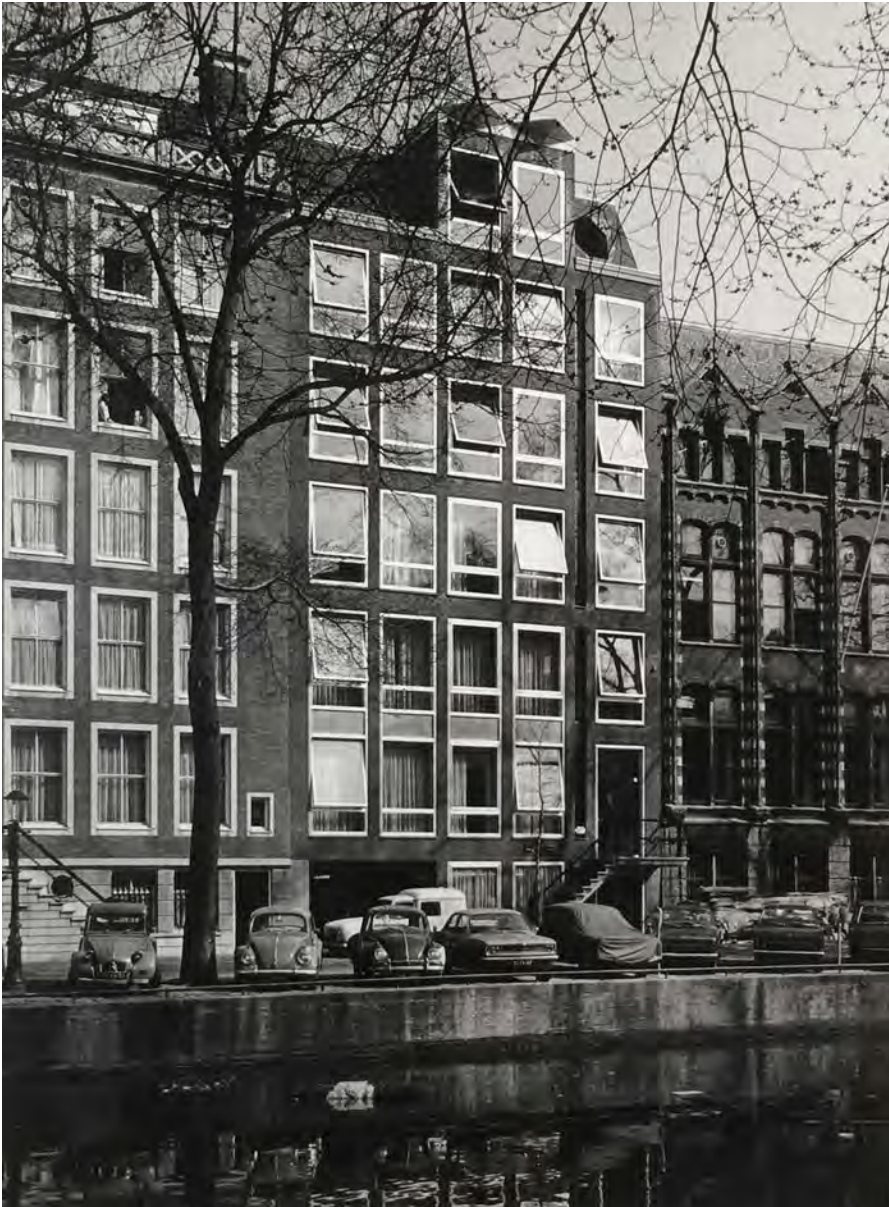
Office building in between canal houses on Keizersgracht (1968), with the pivot windows that gives the facade a very dynamic appearance.
