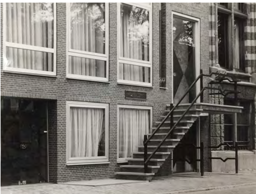
Main entrance stair to the piano nobile with original glass front door and subtle house number 277.
