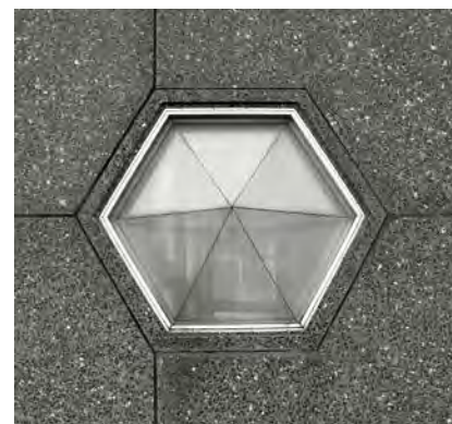
Hexagon window in the gravel concrete ground level underneath the Shell tower in 2012.
