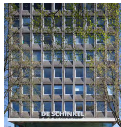
Gravel concrete grid facade in De Schinkel office complex (1968) in 2016. Image: Bart van Hoek.
