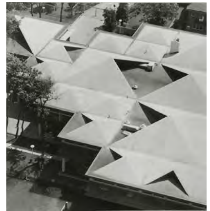
Roof of the Shell canteen (1976) featuring triangular, pyramid-shaped roofstructure.
