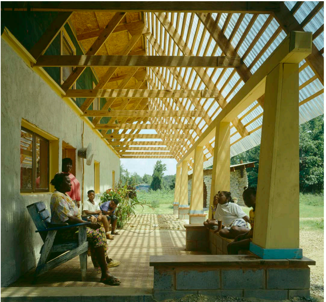
Bryant (Hay Bale) House, the Rural Studio’s first house has walls made of hay bales.
