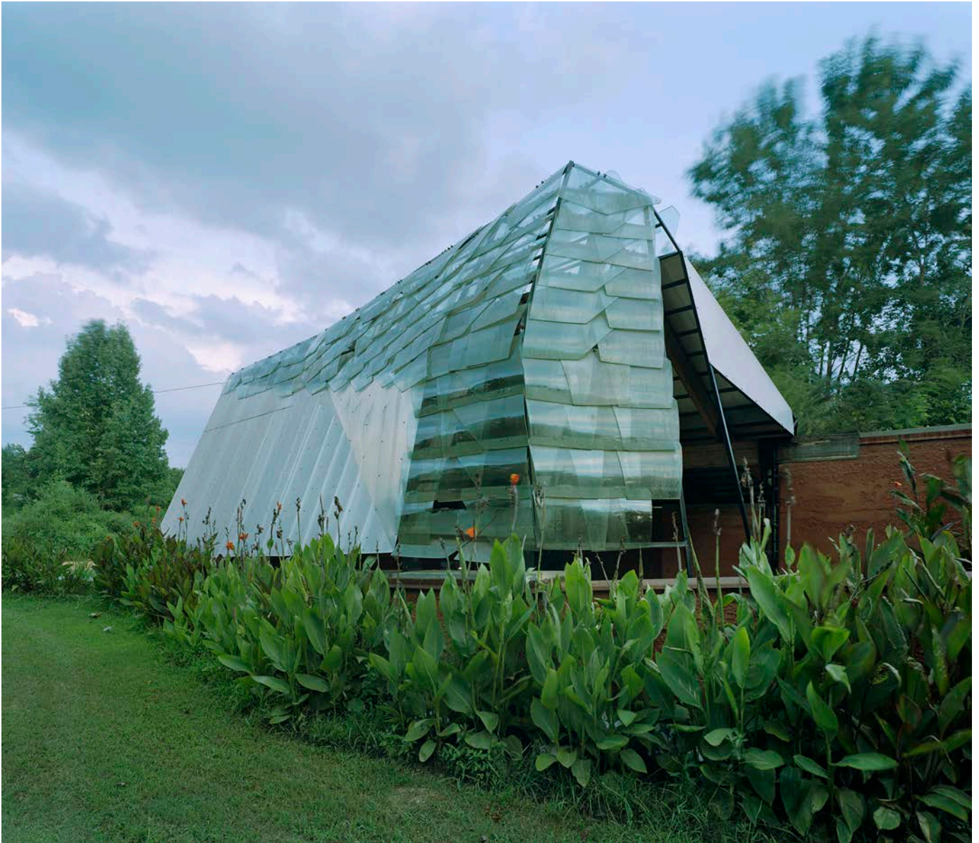
A façade of car windows partially covers a raised nave and aisle.
