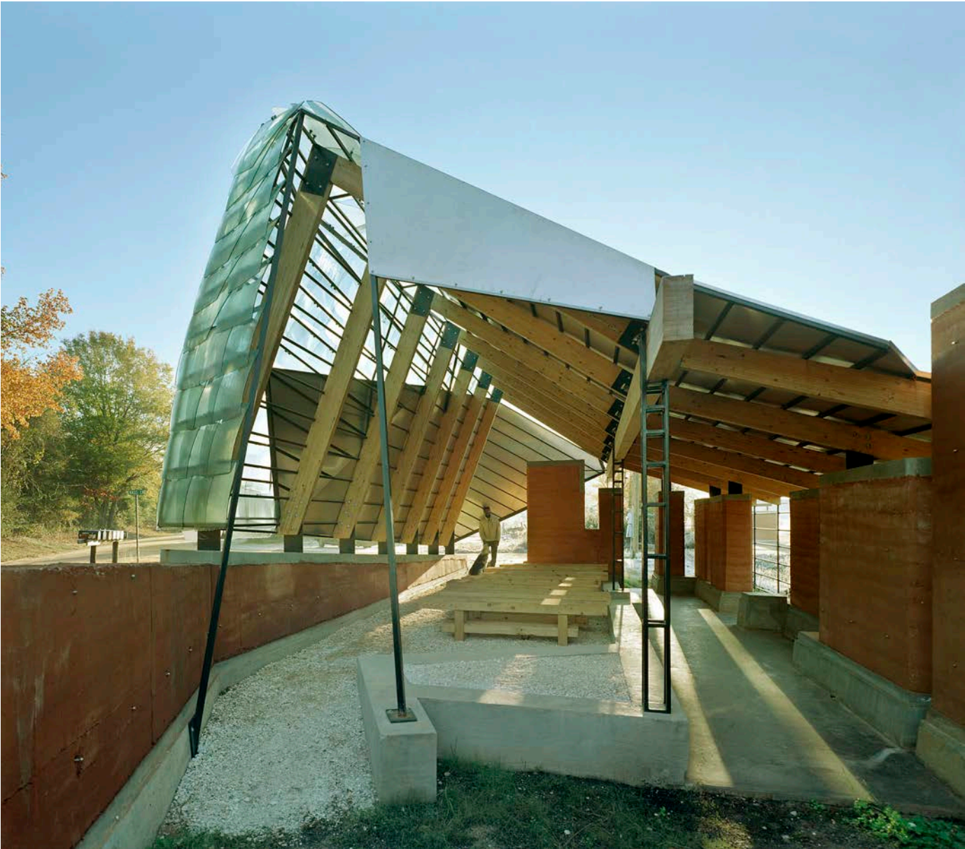
The building leads visitors through a narrow entrance to a space used as a meeting place and chapel.
